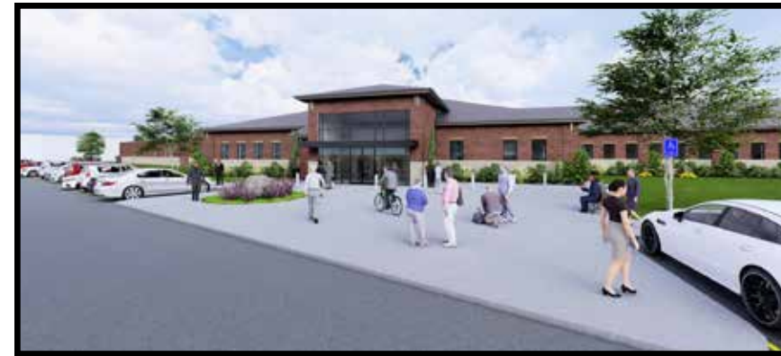
Artist rendering of the new Hamilton Police Department Headquarters set to open in late 2024.
